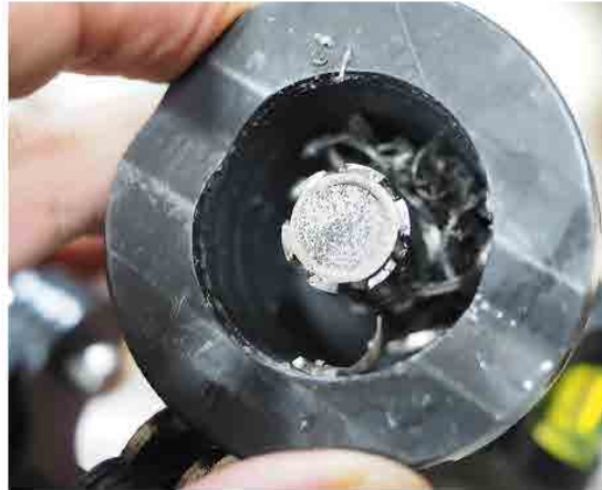
After drilling EACH hole, inspect the cutter assembly. Check for a slug and swarf build up (present in the above image)
